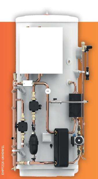
6.0kW & 8.5kW Ecodan are compatible with both variants of 210L cylinder. The 22mm pipework variant is recommended for 6.0kW & the 28mm pipework variant is recommended for 8.5kW.
