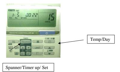
Using the TEMP/DAY buttons advance to code 2C. Using Timer up/down buttons set this to 0002. Press set to register this setting.
