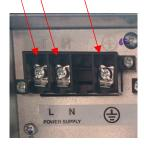
For interconnecting cable (3 core + earth / 4 core) use terminals 1,2 & 3 per set of pipes or indoor FCU used for example our first unit would be unit A and the  $2^{nd}$  Unit being Unit B.
