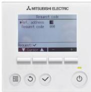
In the Request code screen enter the **outdoor unit address** and the appropriate **rotation setting** see list on reverse.
