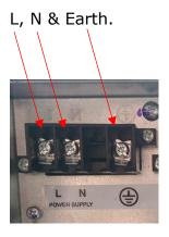
For interconnecting cable (3 core + earth / 4 core) use terminals 1,2 & 3 per set of pipes or indoor FCU used for example our first unit would be unit A and the  $2^{nd}$  Unit being Unit B.
