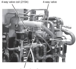
4-way valve coil fixing screw
