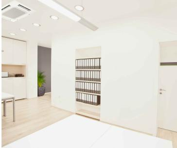
The Mr Slim multi-split system is an ideal option for open plan spaces in medium sized premises such as offices or shops where two units are required. These can be Mr Slim ceiling cassettes (PLA-ZRP) or ducted (PEAD-RP) models and can be connected to a single outdoor unit using twin multi distributor pipes.
